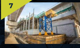
Ongoing foundation works for tower crane at the Metro Prima MRT Station site.
