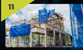
View of ground roof casting for Entrance 1 at the Kampung Batu MRT Station site.
