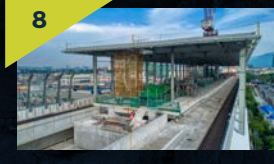
View of the ongoing architectural works such as blockwall, plastering and painting at platform level of the Kepong Baru MRT Station.
