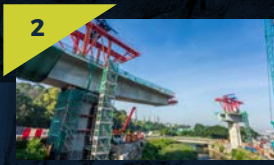
Segmental box girder erection for long span crossing no. 1 in progress at Sungai Gasi near the Sungai Buloh Toll.
