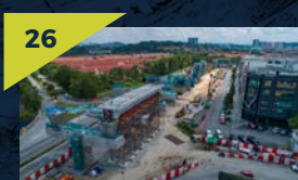
Completion of segmental box girder erection at the Taman Putra Permai MRT Station site.
