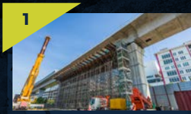
Completion of segmental box girder erection using trestle at the MRT Sungai Buloh-Serdang-Putrajaya (SSP) Line alignment near IGB International School.
