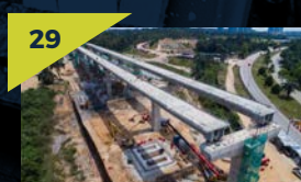
Segmental box girder launching works completed at the Cyberjaya City Centre MRT Station site.
