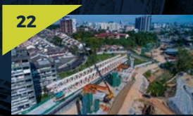
Aerial view of works in progress for station concourse and segmental box girder launching at the Taman Naga Emas MRT Station site.
