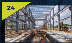
Trenches and slab preparation for concreting at Serdang Depot infrastructure workshop.
