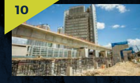
Concourse level beam and slab false-work erection in progress at the Sri Delima MRT station site.
