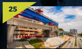
View of the segmental box girder erection at the Equine Park MRT Station site.
