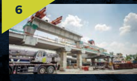
Installation of launching gantry in progress at Kepong Sentral MRT Station site. T-beam installation has been completed for the station's concourse level.
