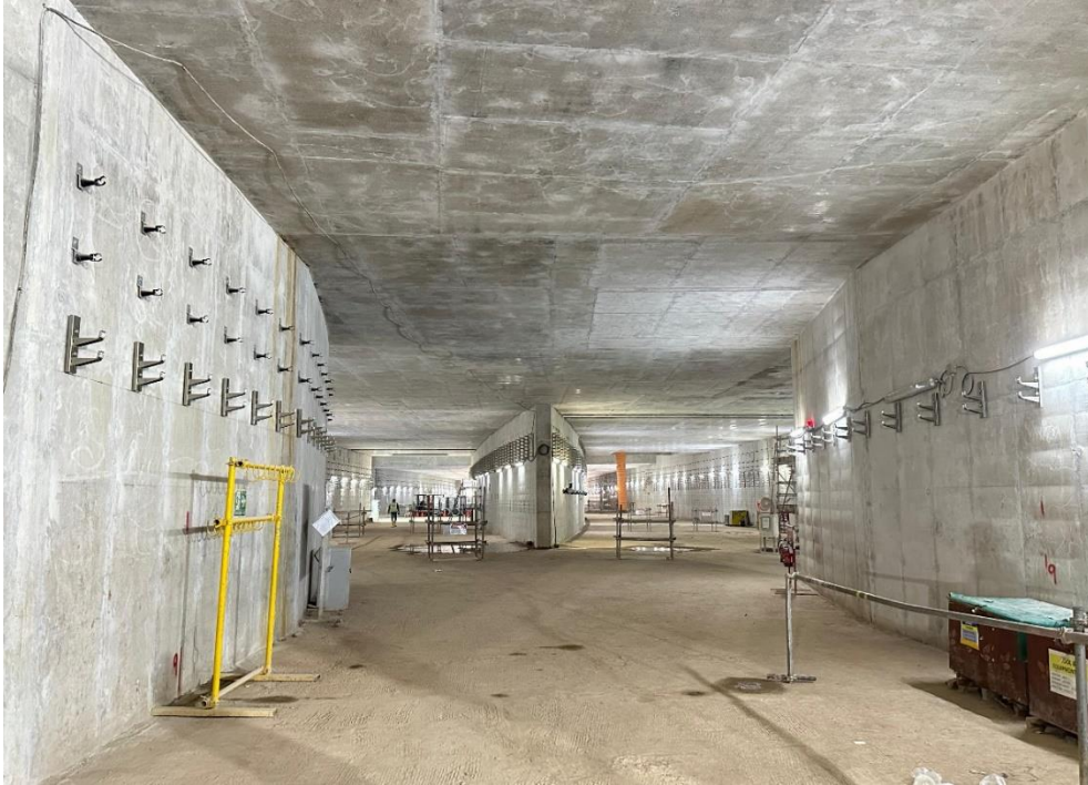
Running Tunnels Box
