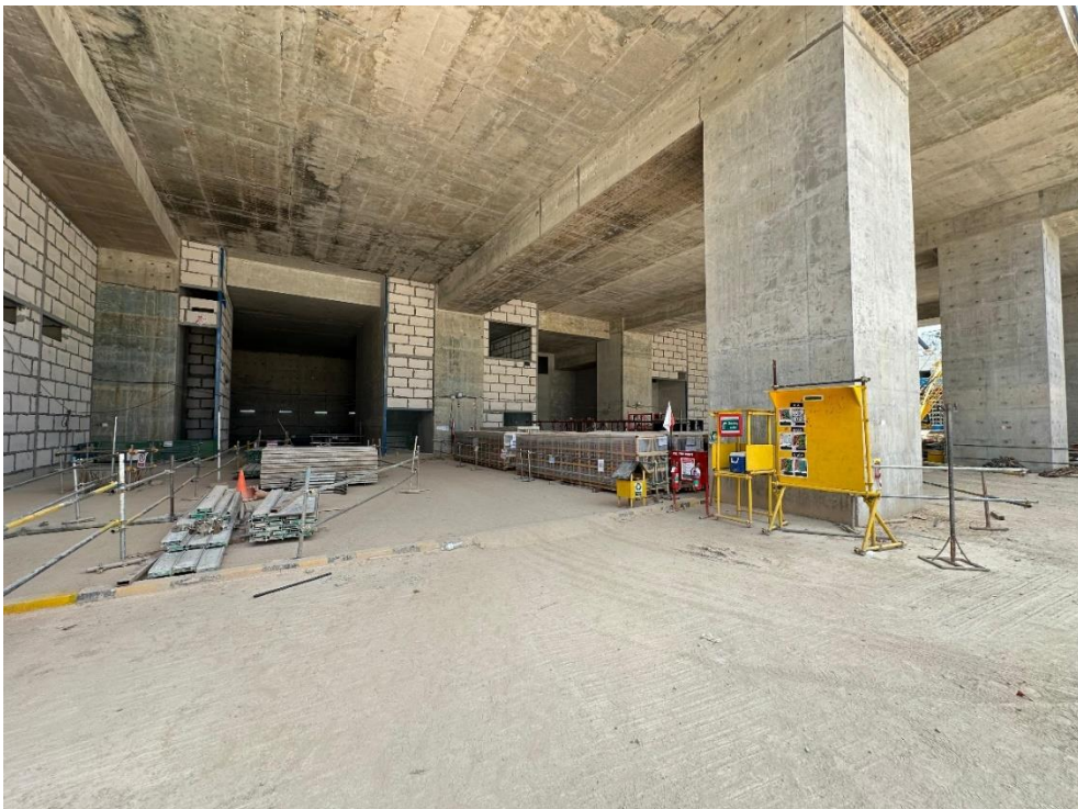
Ticketing Concourse Back of House Civil Structures
