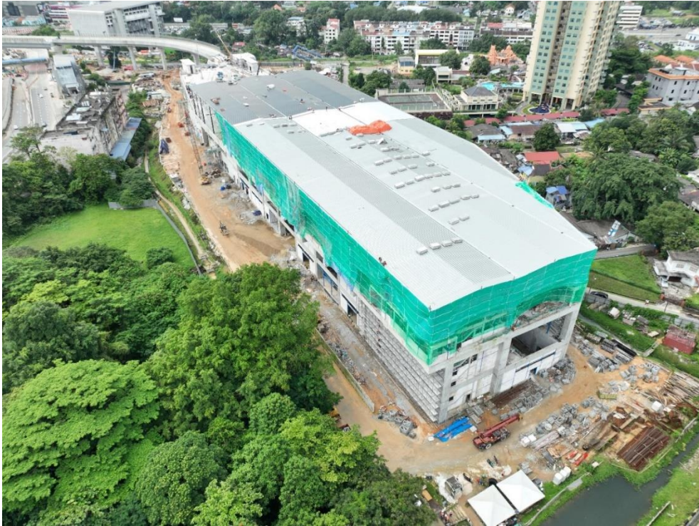
RTS Link Maintenance Depot
