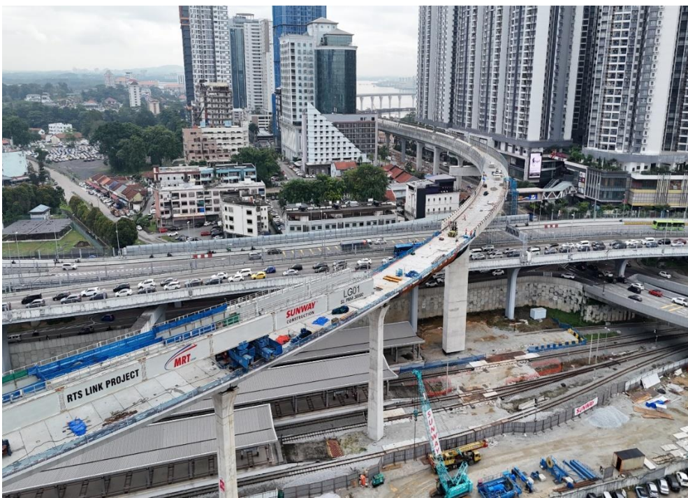
Terrestrial Viaduct along Jalan Tun Abdul Razak
