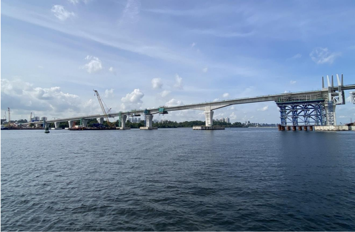
Marine Viaduct Segmental Box Girders fully launched
