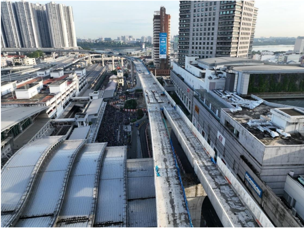
Terrestrial Viaduct along Jalan Tun Abdul Razak
