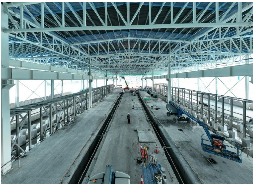
RTS Link Maintenance Depot
