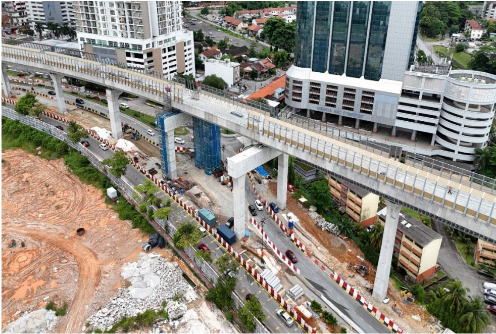
Terrestrial Viaduct along Jalan Ismail Sultan
