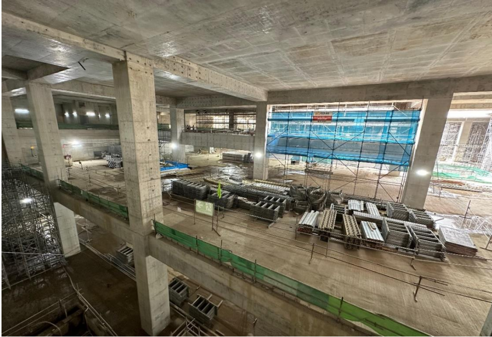
Station Basement 1 and Basement 1 Mezzanine Civil Structures
