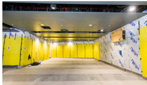
Ongoing cladding works at Conlay MRT Station concourse level.
