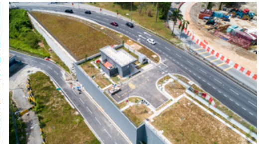
Louvres installation in progress at the Intervention Shaft 1 building structure.
