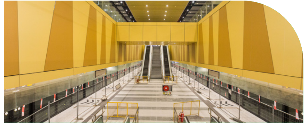
Completed finishes at the concourse and platform levels of the Raja Uda MRT Station.
