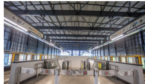
Escalator barrier completed at the platform level of the Cyberjaya Utara MRT Station.
