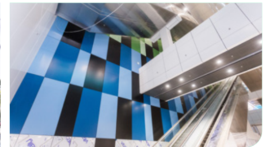
Architectural finishes for the lower platform level of the Ampang Park MRT Station.
