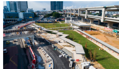
Covered walkway at the Chan Sow Lin MRT Station.
