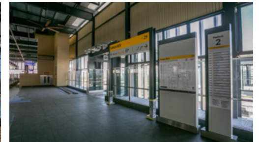
View of the completed installation of directional signages, information board and integrated map at the Sungai Besi MRT Station.
