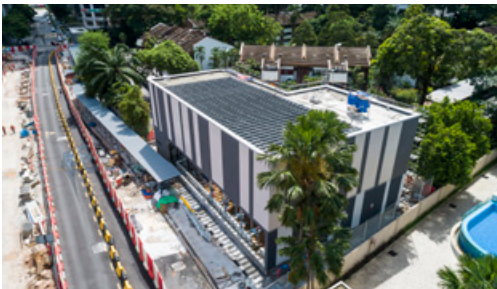
Overall view of the Persiaran KLCC MRT Station Cooling Tower.
