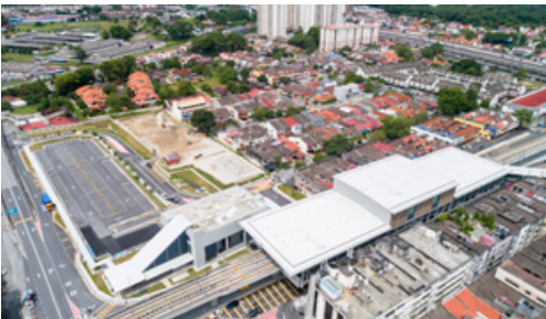
Defects rectification works in progress at the Kentonmen MRT Station.
