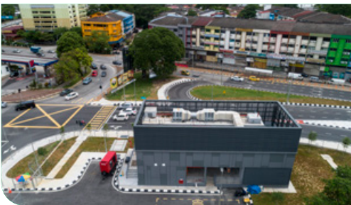
Overall view of the completed Escape Shaft 1, along Jalan Sultan Azlan Shah.
