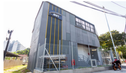
View of the Escape Shaft 2 building from ground level.
