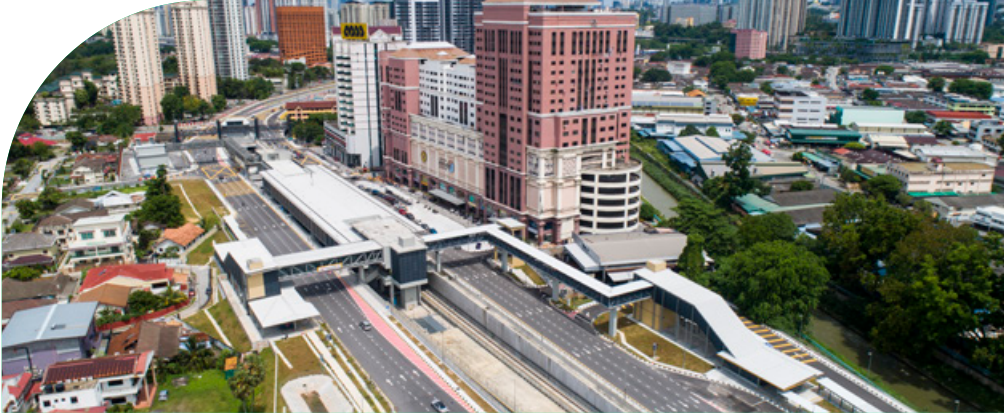
Defects rectification works in progress at the Jalan Ipoh MRT Station.
