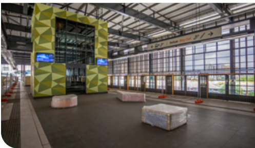
The platform benches were delivered and positioned at the Kuchai MRT Station.
