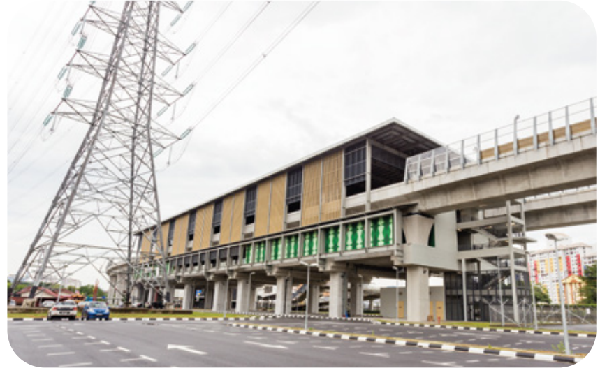
View of the Kampung Batu MRT Station.
