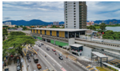
Aerial view of the Sri Delima MRT Station.
