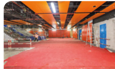
Aerial view of the Conlay MRT Station showing the backfilling works in progress.
