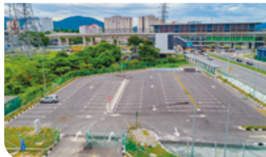
At-grade park and ride of Jinjang MRT Station.
