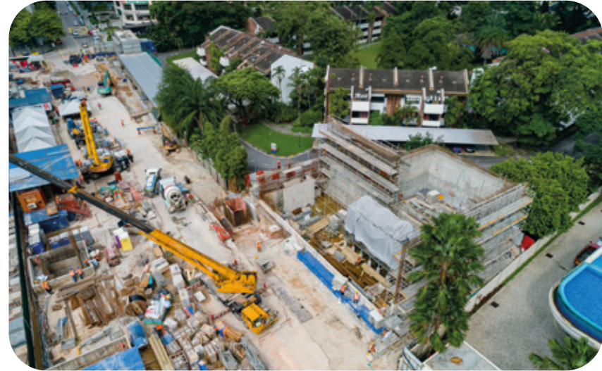
Overall view of the Persiaran KLCC MRT Station construction site.
