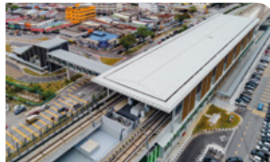
View of the Kepong Baru MRT Station.
