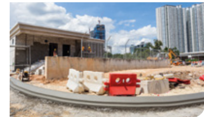
Road kerb construction works in progress at the South Portal.
