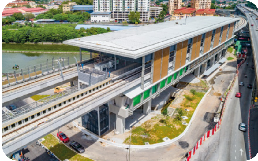
Aerial view of the Sri Damansara Timur MRT Station.
