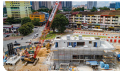
Aerial view of the Escape Shaft 1.
