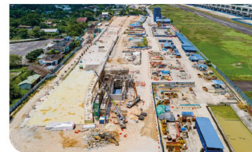
Aerial view of the Bandar Malaysia Selatan MRT Station.
