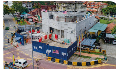
External plastering and installation of groove line at the Escape Shaft 2.
