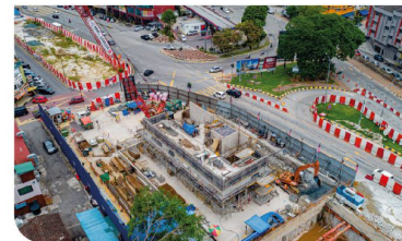
Aerial view of the Escape Shaft 1 with 84% progress completion.
