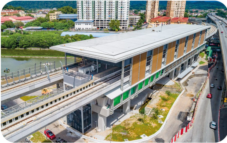
Aerial view of the Sri Damansara Timur MRT Station showing the site preparing for BOMBA inspection.
