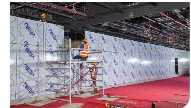
Cladding installation works at the Titiwangsa MRT Station concourse level.
