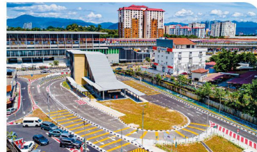
Aerial view of the Kepong Baru MRT Station showing the road and drainage works completed and inspected by Dewan Bandaraya Kuala Lumpur.
