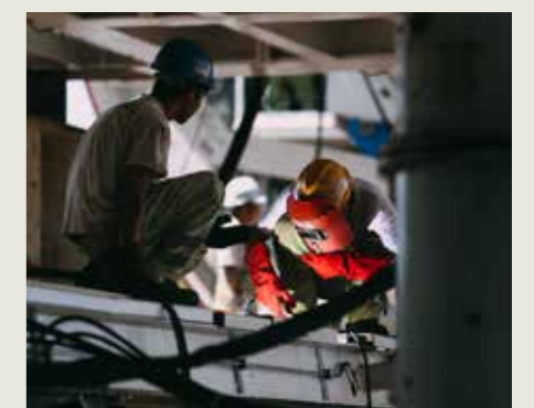
■ AT THE FACTORY: Workers at the Herrenknecht Tunnelling Machinery Co. Ltd. in Guangzhou, China working on the Tunnel Boring Machines.
