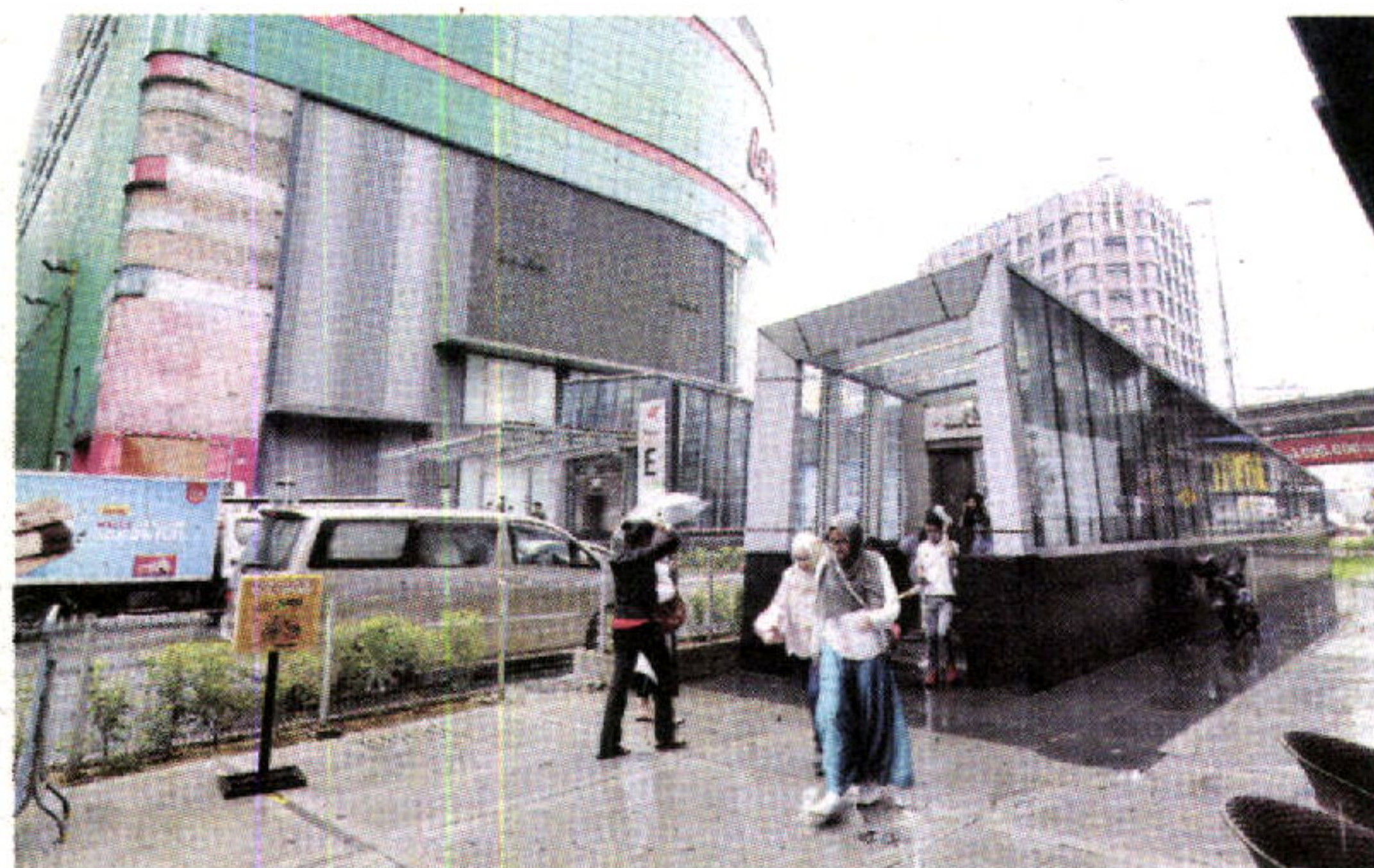
The façade of Entrance E.
