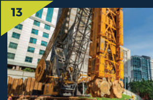
Diaphragm wall construction ongoing at the Ampang Park MRT Station site.
