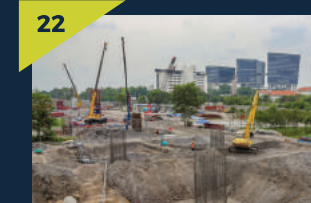
Pile cap works in progress at the Putrajaya Sentral Station site.
