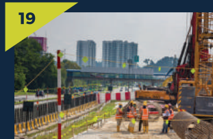
Bored piling works in progress at the Equine Park Station site.
