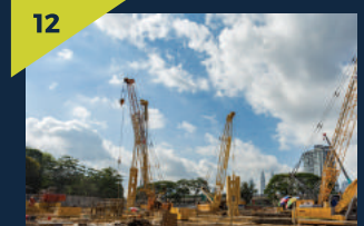
Foundation for the chiller plant being built at the Titiwangsa Station site.
