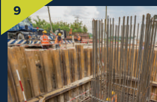
Pile cap works in progress at the Sri Delima Station.
