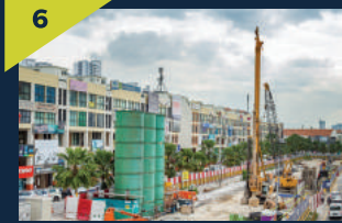
Bored piling works in progress at the Metro Prima Station site.
