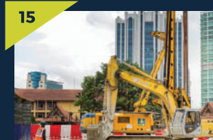
Ongoing secant bored pile works within the Conlay Station site.
