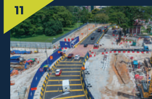
Road diversions on Jalan Sultan Azlan Shah for the construction of the Sentul West Station.
