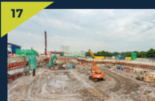
Station box excavation works at the Bandar Malaysia North Station site.
