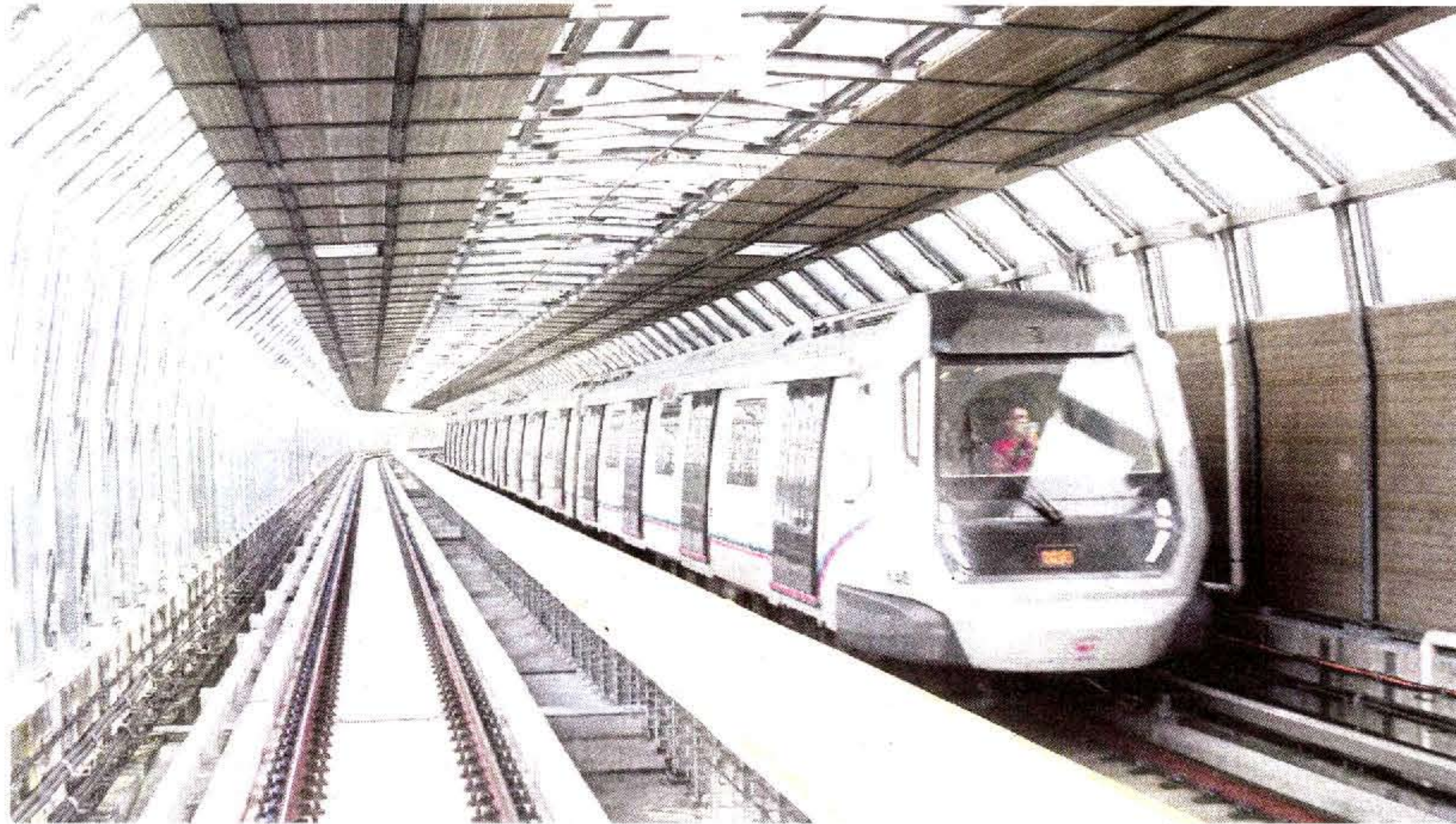
The Mass Rapid Transit Sungai Buloh-Kajang Line is said to be on a par with the New York City Subway or London Underground public rapid transit system. FILE PIC
