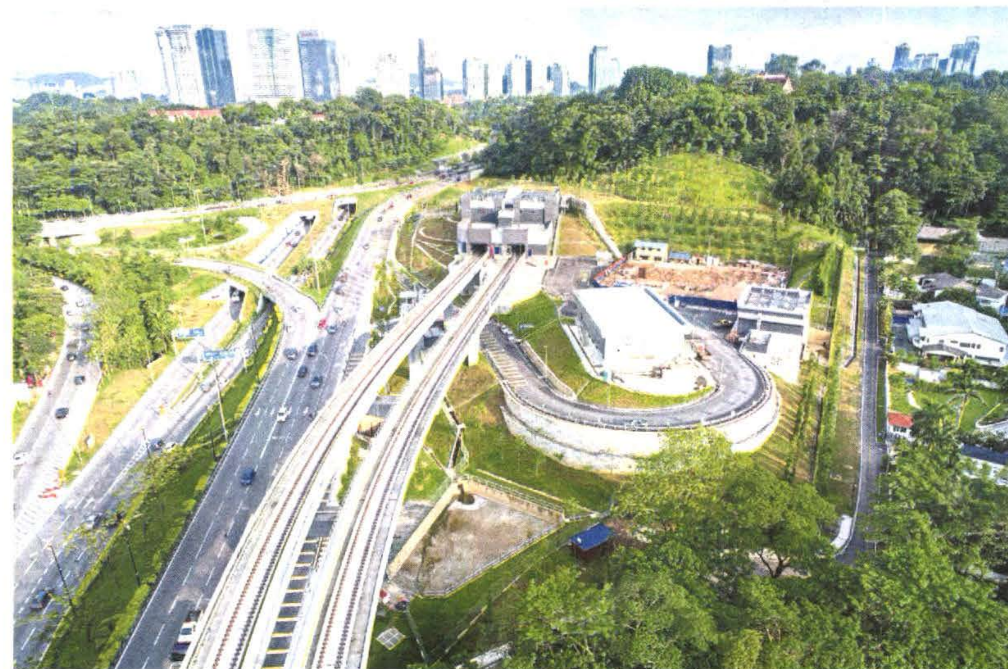
Seen here against the backdrop of the Kuala Lumpur city skyline is the Semantan North Portal, which is the interfacing point between the underground track and the elevated track of the KVMRT Sungai Buloh-Kajang line.
