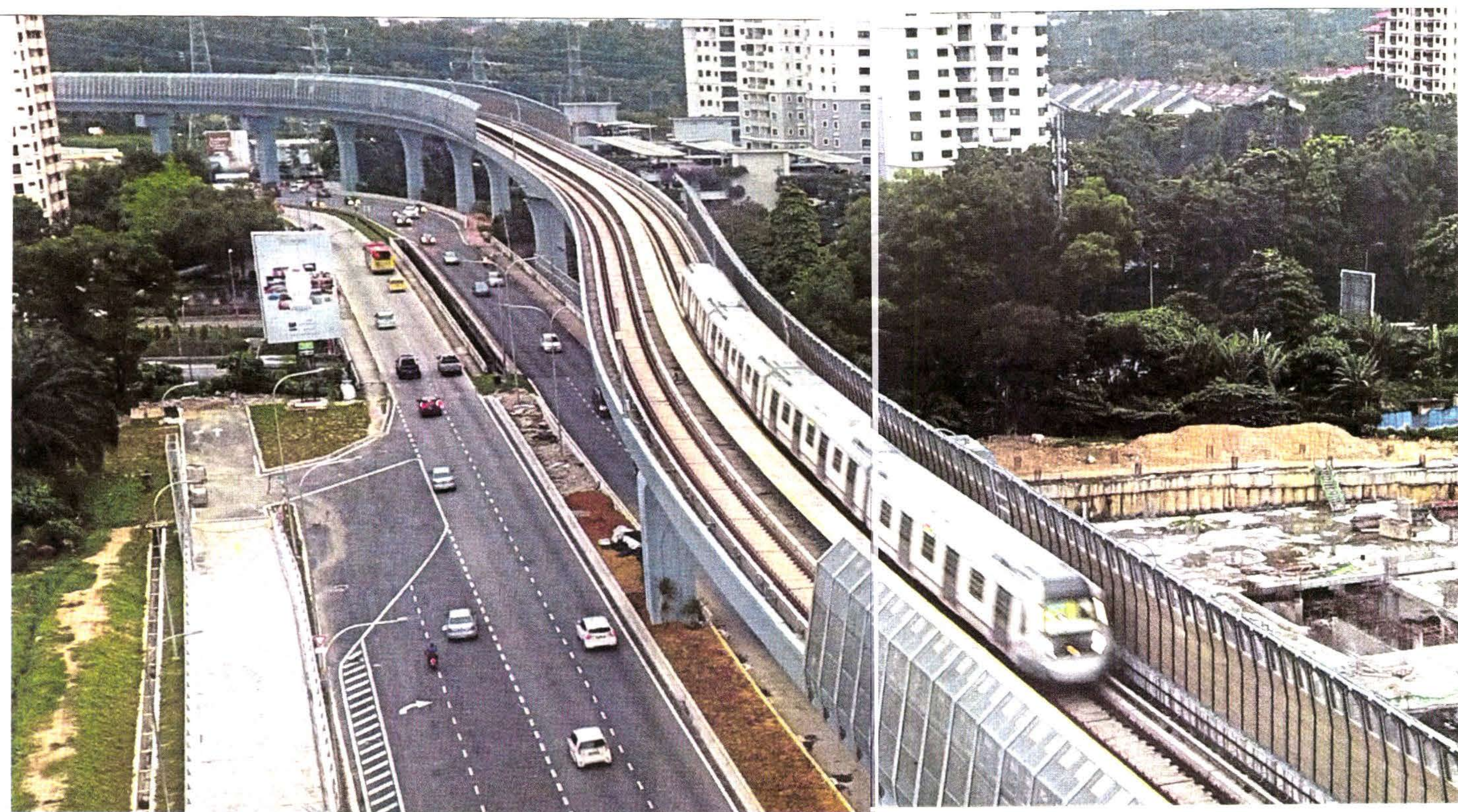
A test run of the MRT train at Sunway Damansara in Petaling Jaya yesterday. Pic by Zunnur Al Shafiq
