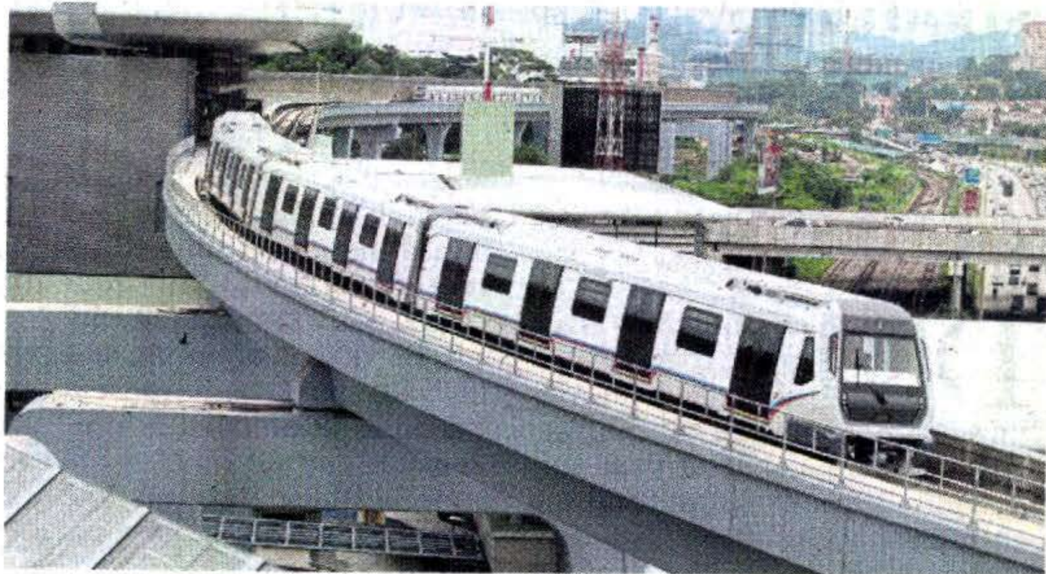
A Mass Rapid Transit train being tested at the Sungai Buloh station. File pic
