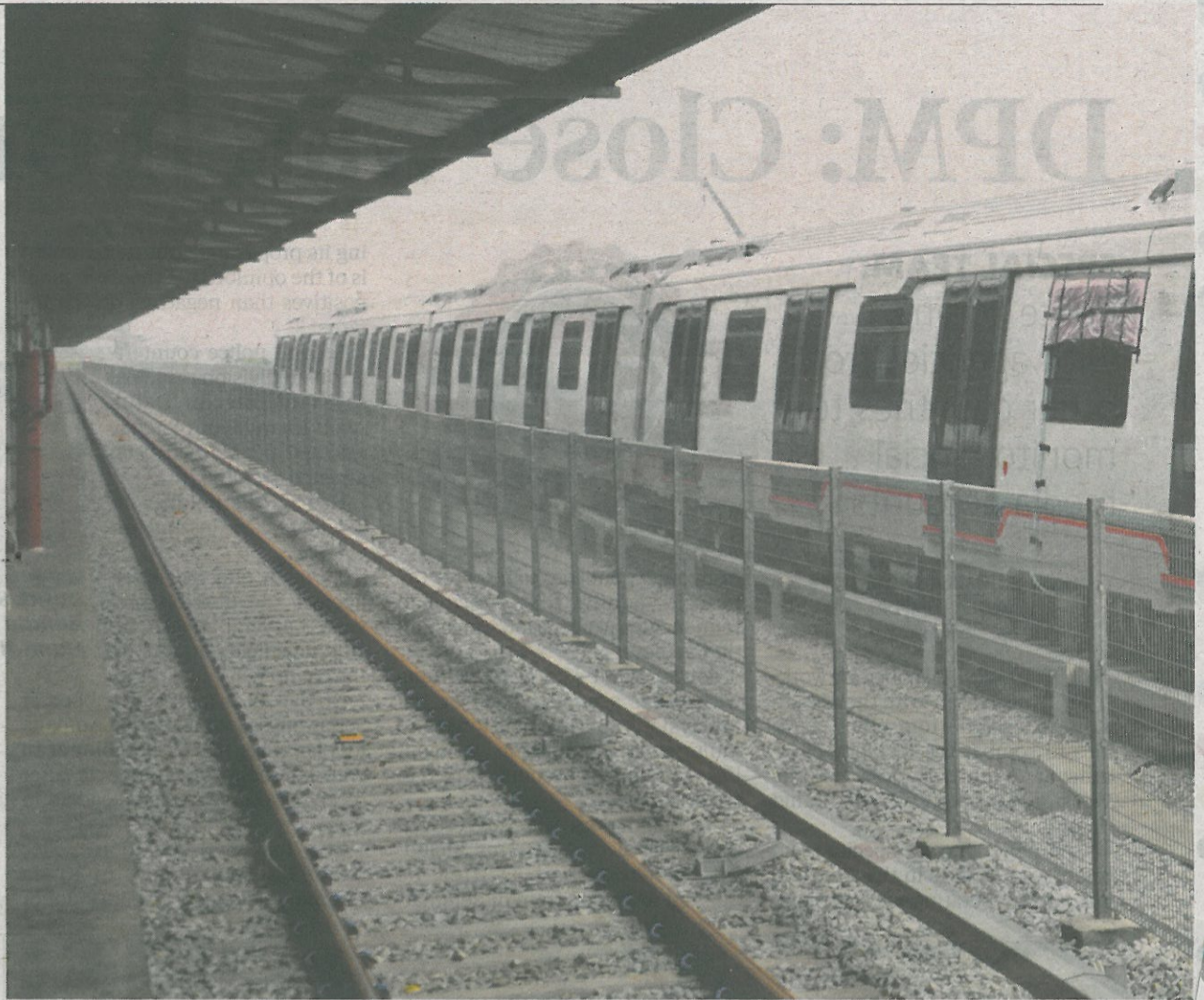
The Project Development Partner concept adopted for the MRT project eliminates risk of cost overrun and ensures quality of work.
