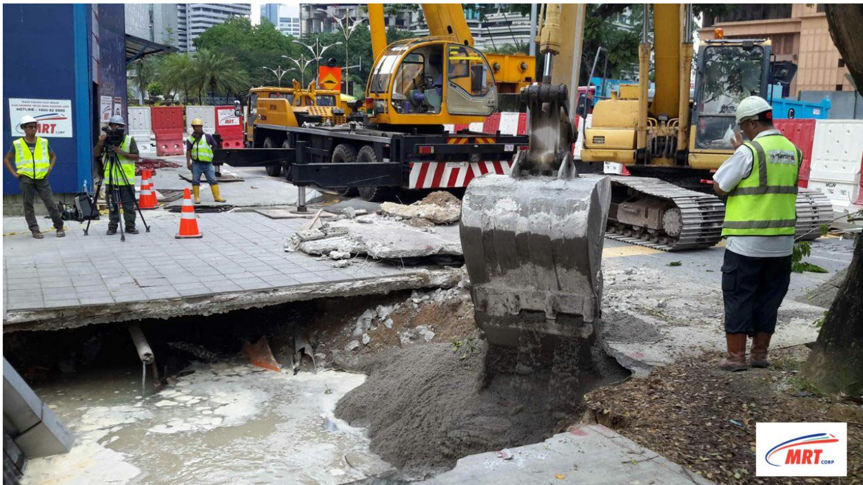
Backfilling of the sinkhole in progress.
