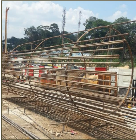
A side view of the rebar cage that was being fabricated.
