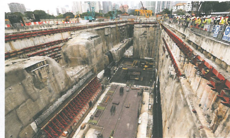
MRT works in progress ... Line 2 is targeted for completion in 2022
