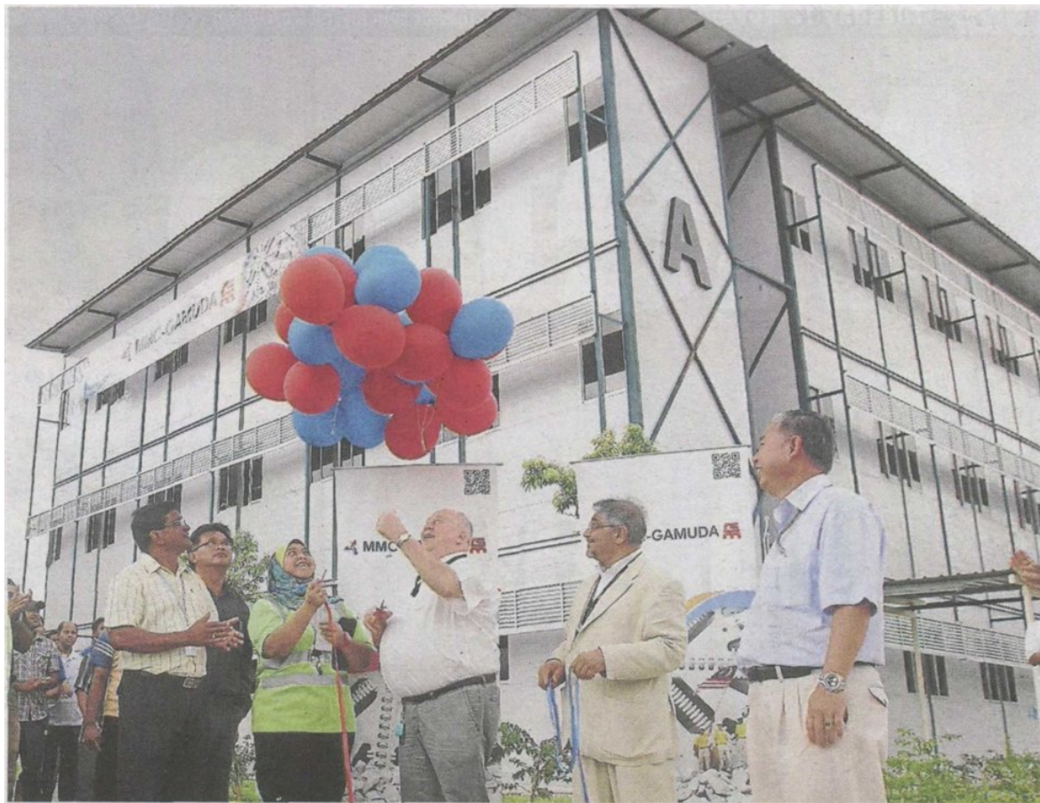
New start: (From right) MGKT head of plant and machinery and store Hong Fook Main, Satpal, MGKT project manager Gustav Klados and CLQ manager V. Visvanathan (left) during the opening of the new CLQ.
