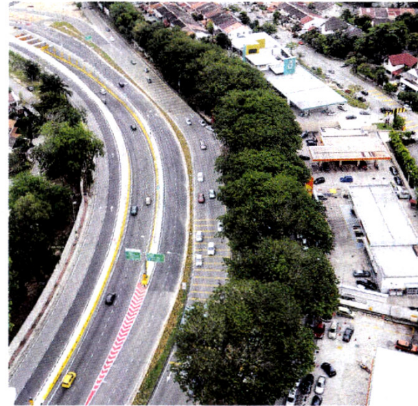
TOO CLOSE: The proposed MRT line will be between 14.5m and 15.9m from some of the houses at Pinggir Zaaba — Pix: SHAHIR OMAR
