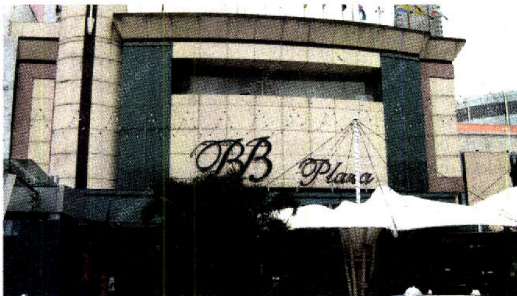
GOING DOWN: The front view of BB Plaza that is due for demolition
