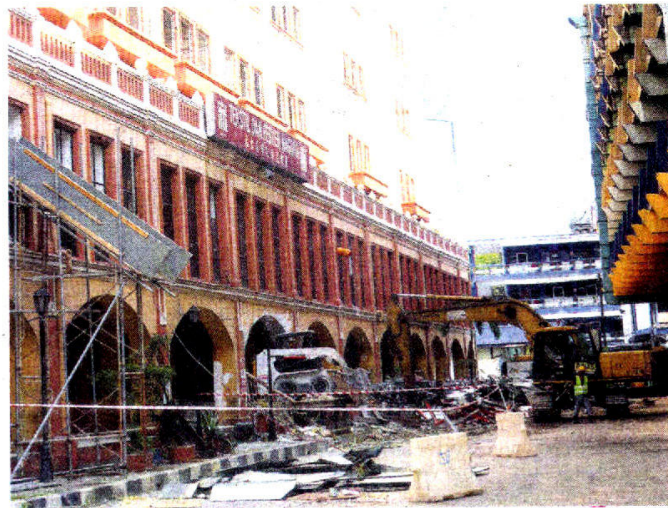
Making way: Uda Ocean demolished for the MRT project.
