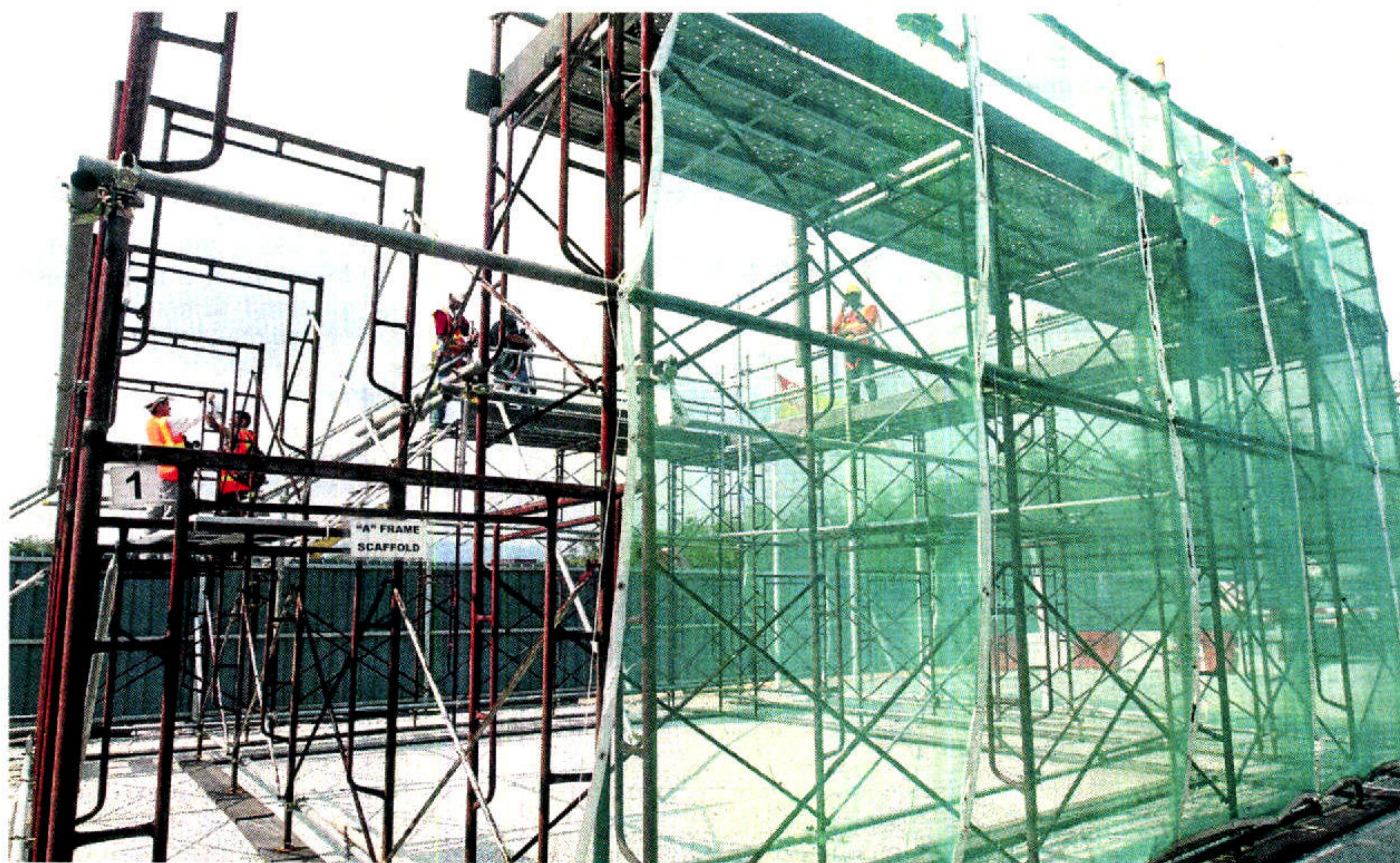
'A' frame scaffold demonstration by MMC-Gamuda workers at the display centre. Pix by Mohd Yusni Ariffin
