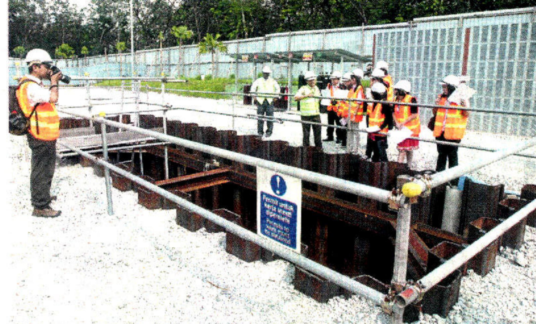
An excavation trench with guard rail.
