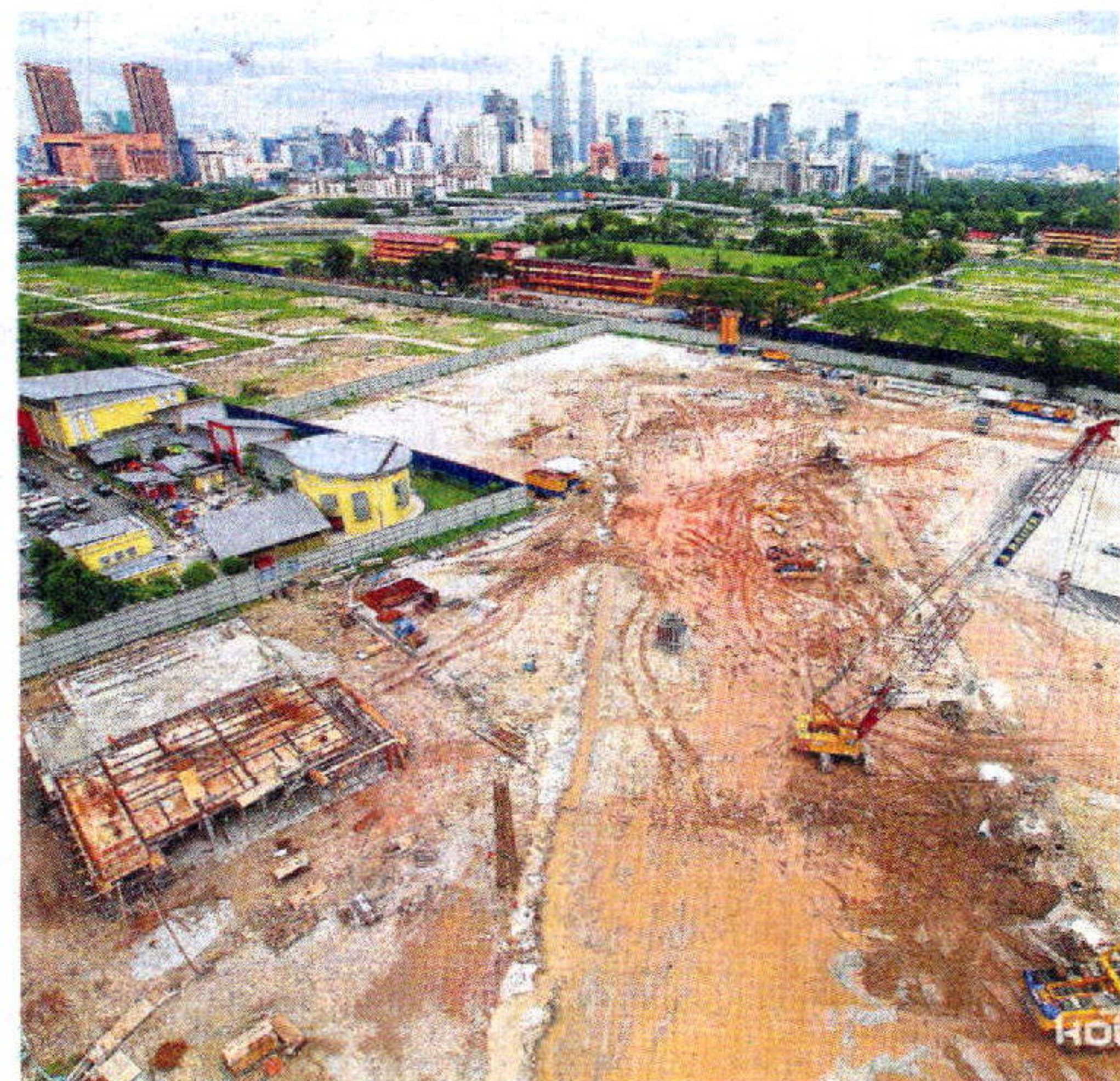
Under way: Construction progress for the Cochrane MRT Station.
